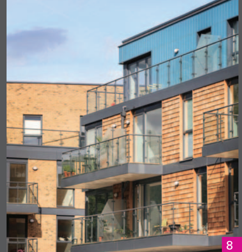
Gunmakers Wharf, Tower Hamlets
